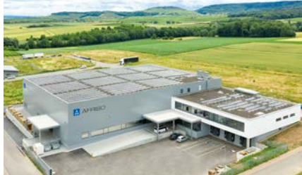
AFRISO logistics and service centre
