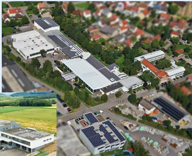
Headquarters in Güglingen (Germany)
