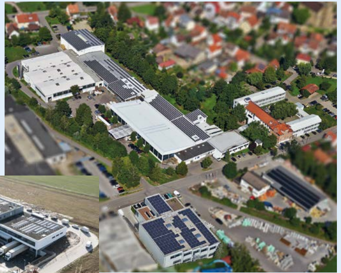
Headquarters in Güglingen (Germany)
