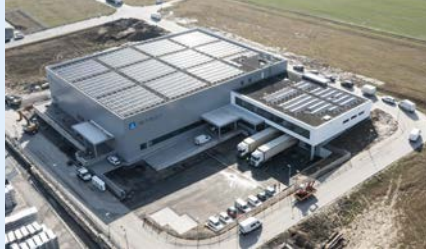
AFRISO Logistics and service centre
