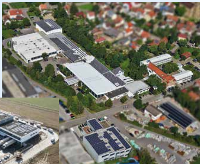
Headquarters in GÜGLINGEN (Germany)
